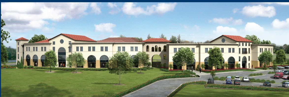
View from West-Parker Coliseum showing future position of building at right.
